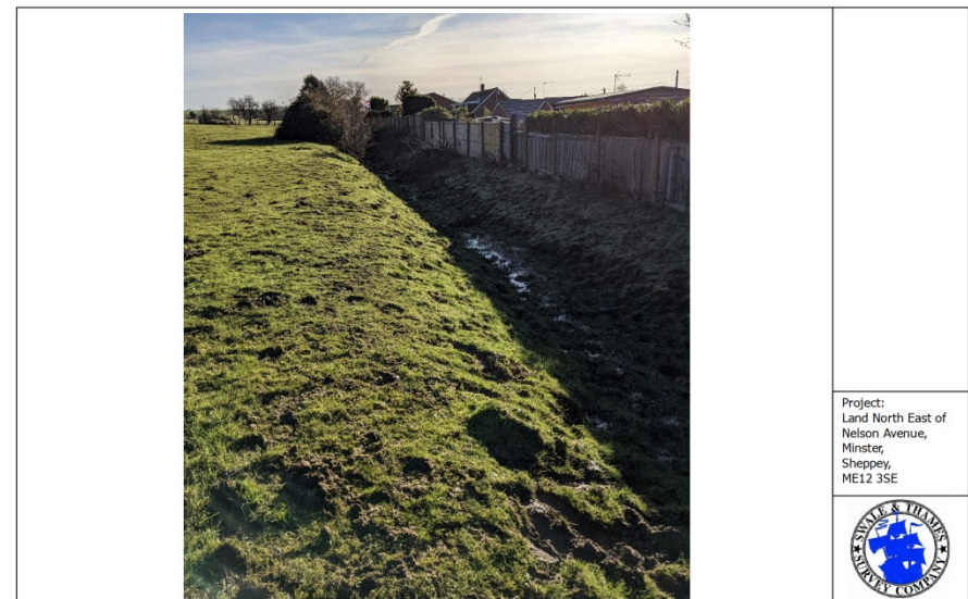
Plate 9: View along the drainage ditch at the southern boundary (facing ESE).
